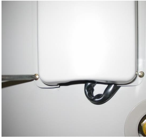
Step 2 remove screws from lower front cover
