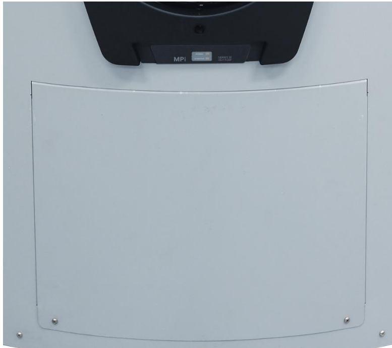
Step 27 replace heat pump module front cover
