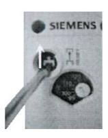
3. Replace high limit reset lever screw cap.
