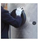
The aluminium disk may be supplied in one piece or two semi circles depending on the tank size. Fit on top of the insulation.
