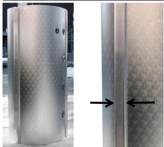
Continue using the same process to wrap each panel around the tank. Once all panels are joined each panel should be tightened into the last tooth if possible. Ensure the teeth are fully engaged along the entire length.
