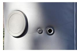
There are 14 plastic fitting surrounds, these vary in size and should fit tightly around the fitting. The fitting surrounds are placed on after the insulation and should sit flush with the front of the fitting. Attach the fitting surrounds as each section is put in place, this will help to hold the section in the correct position as each is added.
