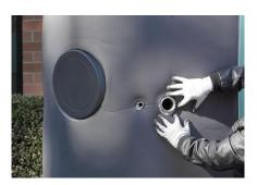
Line up the section that has the two larger holes with the flanges on the tank. The bottom of the insulation should be touching the ground. If there are further holes in the section fit them over the fittings ensuring the insulation is clear of the fittings.
