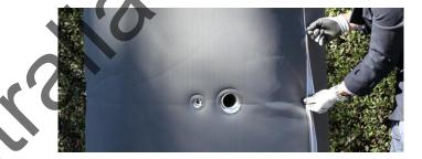
When the first panel is in place, fit the section to the left using the same process. Where the sections meet zip together. Make sure to relieve the stress from the zipper by pulling in the two sections either side of the zipper. We recommend two people to complete this step. **Note: failure to observe this precaution may result in damage to the zipper / insulation.**
