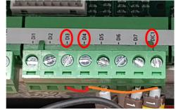
In 4<sup>th</sup> heat pump enclosure: Connect "DI3" with "DI4" and "DIC1". Connect "DIC1" with the existing wire as shown in the picture.
