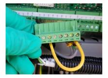
In 3<sup>rd</sup> heat pump enclosure: Connect "DI4" with "DIC1". Connect "DIC1" with the existing wire as shown in the picture.
