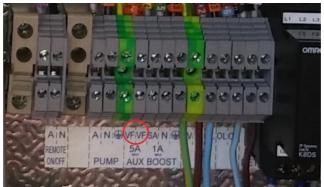
Picture of heat pump terminal strip
