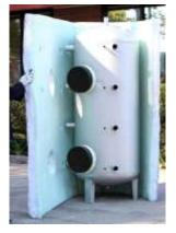
Fit the two green foam insulation rings around the upper and lower flange. Fit the two black plastic flange covers over the foam ring.
