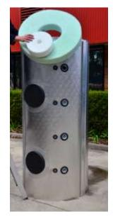
There are two round pieces of insulation that fit on top of the tank. The smaller white high density foam piece fits over the top fitting and the larger green piece fits around the white piece.
