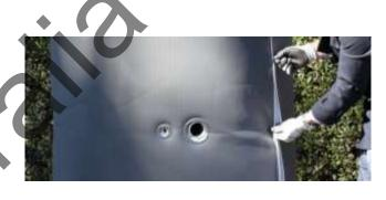
There are 14 plastic fitting surrounds, these vary in size and should fit tightly around the fitting. The fitting surrounds are placed on after the insulation and should sit flush with the front of the fitting. Attach the fitting surrounds as each section is put in place, this will help to hold the section in the correct position as each is added.
