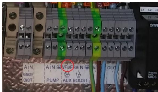
Picture of heat pump terminal strip
