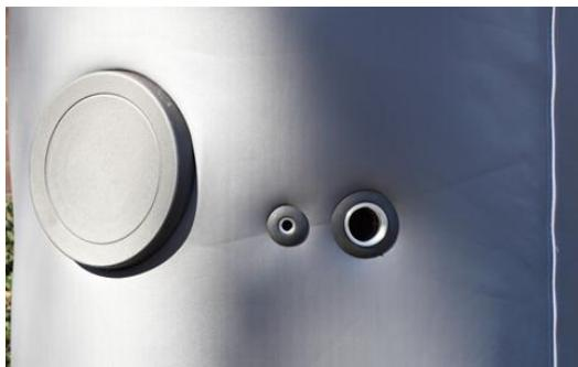
There are 14 plastic fitting surrounds, these vary in size and should fit tightly around the fitting. The fitting surrounds are placed on after the insulation and should sit flush with the front of the fitting. Attach the fitting surrounds as each section is put in place, this will help to hold the section in the correct position as each is added.
