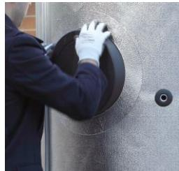
The aluminium disk may be supplied in one piece or two semi circles depending on the tank size. Fit on top of the insulation.
