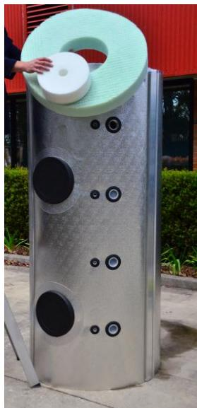
Continue using the same process to wrap each panel around the tank. Once all panels are joined each panel should be tightened into the last tooth if possible. Ensure the teeth are fully engaged along the entire length.
