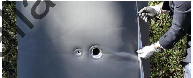
When the first panel is in place, fit the section to the left using the same process. Where the sections meet zip together. Make sure to relieve the stress from the zipper by pulling in the two sections either side of the zipper. We recommend two people to complete this step. **Note: failure to observe this precaution may result in damage to the zipper / insulation.**
