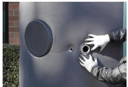
Ensure the drain is fitted or plugged. Ensure the tank is in position where it's going to be installed, as it can be difficult to move once the insulation is attached.
