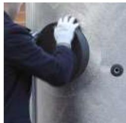
The aluminium disk may be supplied in one piece or two semi circles depending on the tank size. Fit on top of the insulation.
