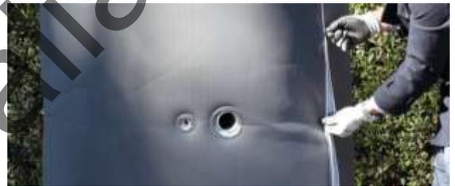
There are 14 plastic fitting surrounds, these vary in size and should fit tightly around the fitting. The fitting surrounds are placed on after the insulation and should sit flush with the front of the fitting. Attach the fitting surrounds as each section is put in place, this will help to hold the section in the correct position as each is added.
