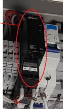
The phase detect relay will open circuit if the heat pump has been wired with incorrect phase rotation or if a phase has failed. Both red and green LEDs on the relay will be illuminated if phase rotation is correct.
